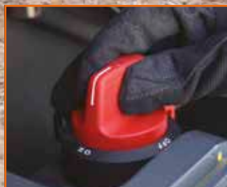
Battery cut-off switch
